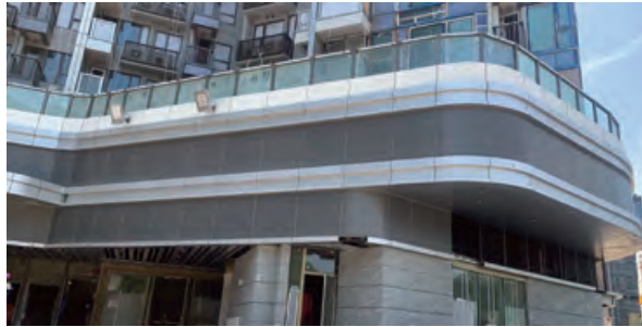
Residential development at Site A and Estate Road of Wong Chuk Hang Station property development, Aberdeen Inland Lot No. 467 香港仔內地段第467號黃竹坑站物業發展項目及地盤A
